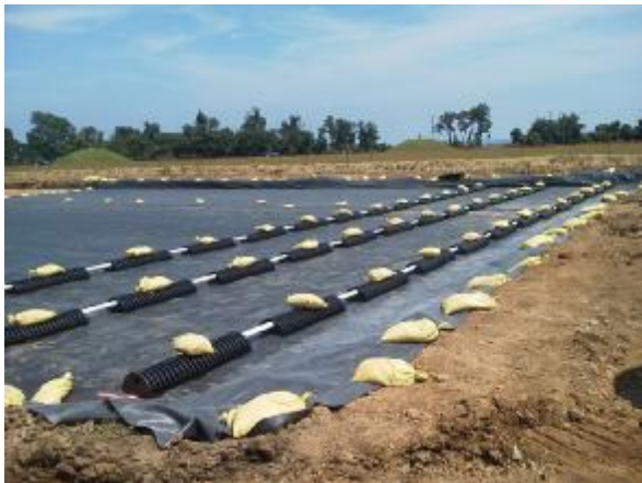
Placement of Firestone EPIC Chambers
