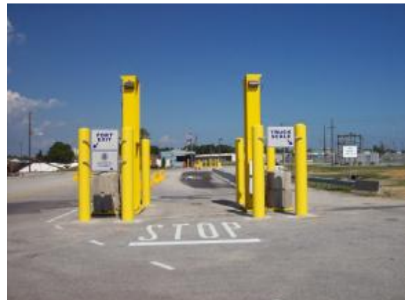
Secondary RPM Installation
