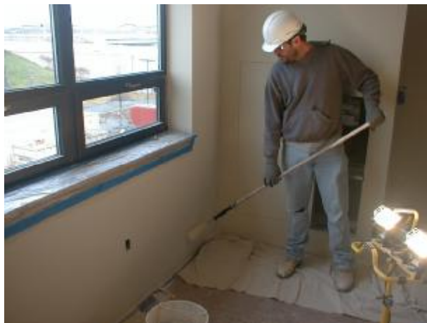
Painting the Replaced Wallboard
