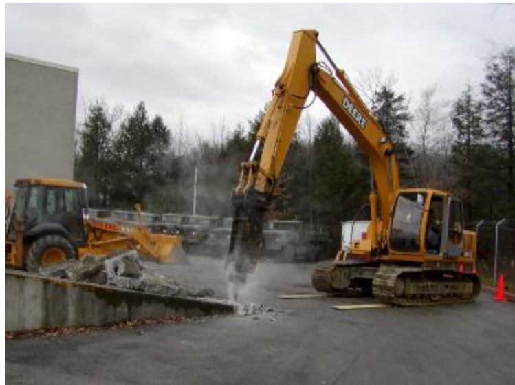
Demolition of Concrete Ramp
