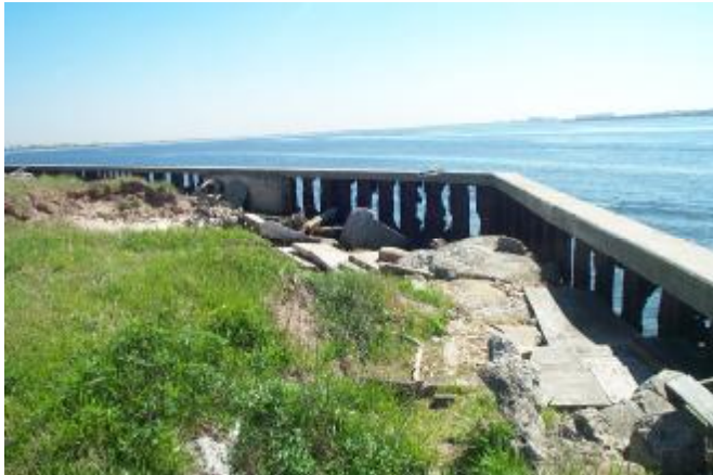
Old Sheet Pile Seawall
