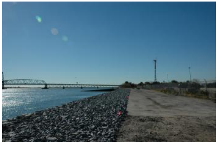
New Revetment Seawall
