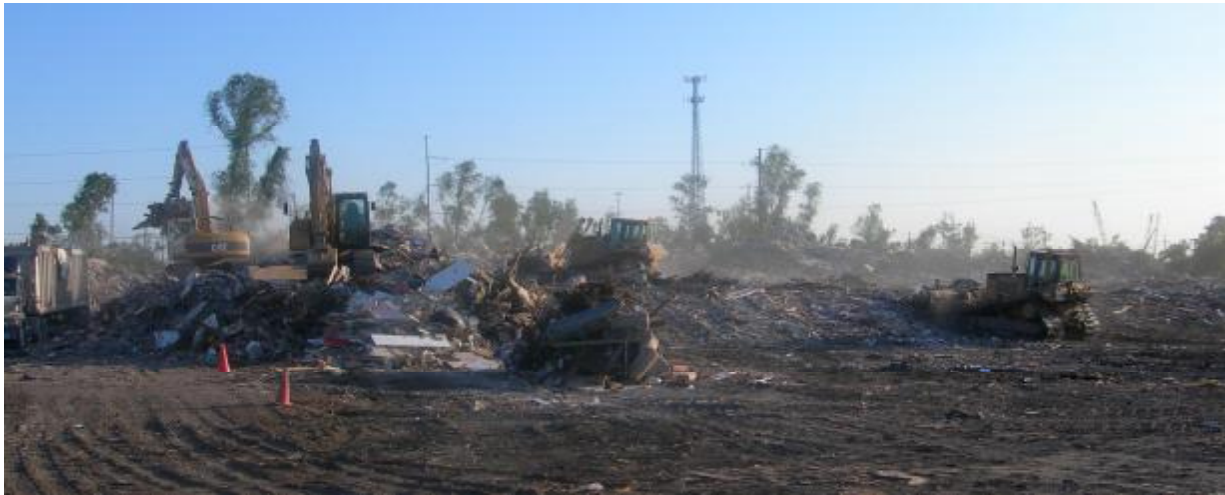
Peters Road Dump Site Operations
