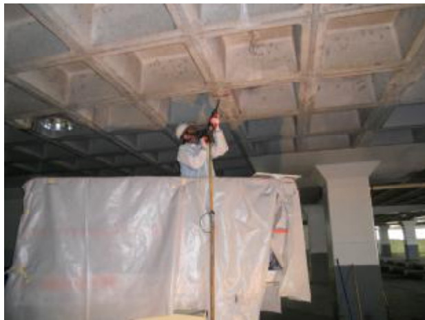
Removing Contaminated Concrete
