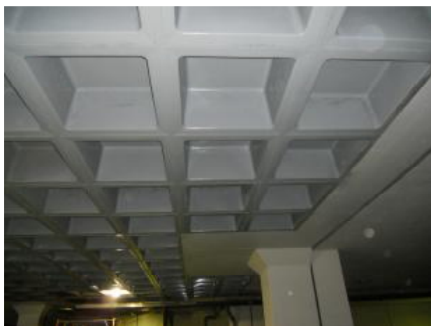
Repaired and Encapsulated Concrete
