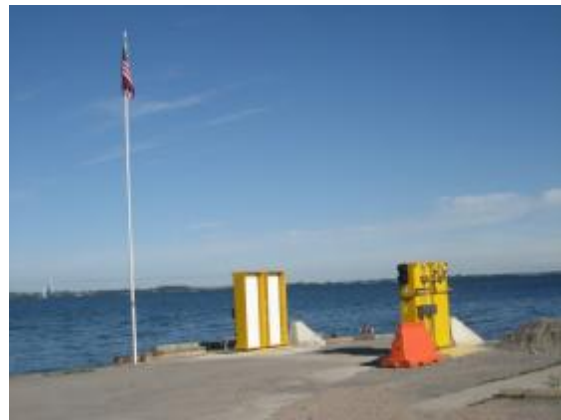
Completed RPM Installation
