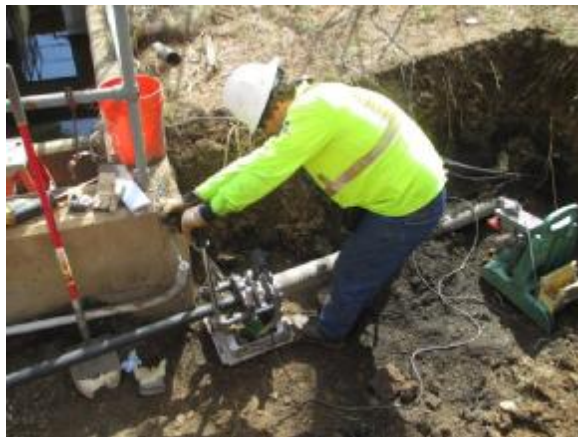
Fusion Welding Dual-Walled Piping
