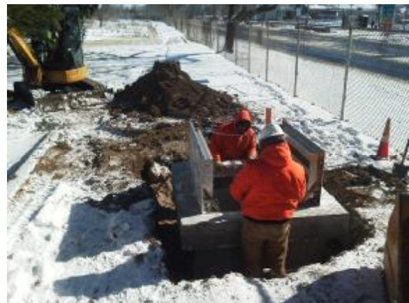
Installing New Well Vault
