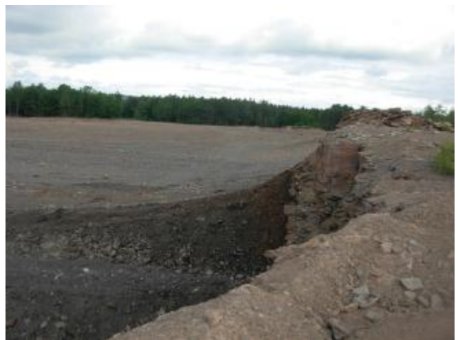
Filling in strip pits
