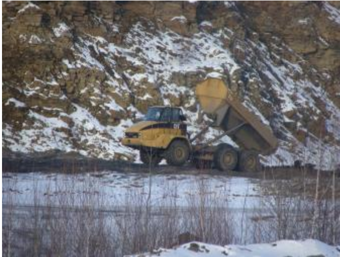
Relocating fill material via dump truck
