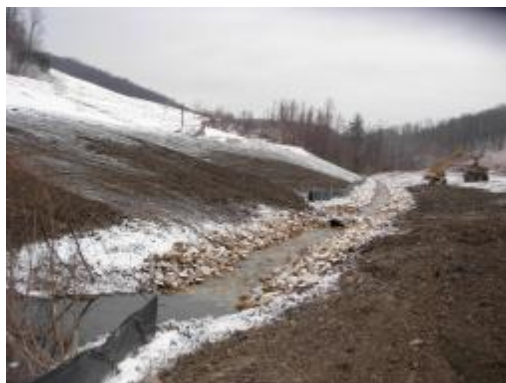
Grading and Constructing the Swale
