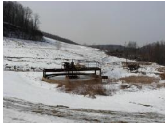
Initial Site Conditions
