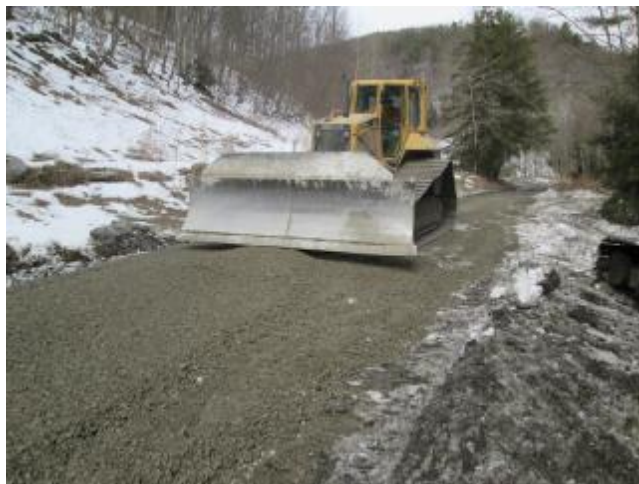
Grading stone surface
