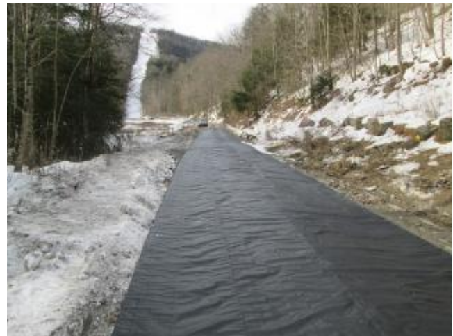
Placing geotextile fabric
