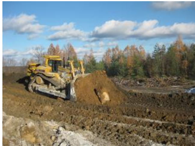
Grading and incorporating alkaline material
