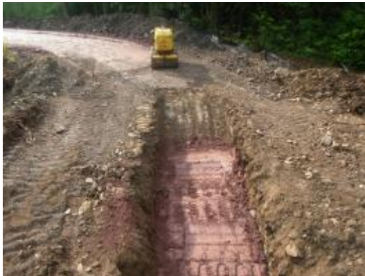
Constructing the Cut-Off Trench
