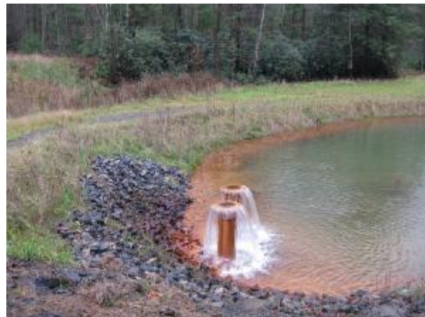
Settling Pond with Inlet Aerators
