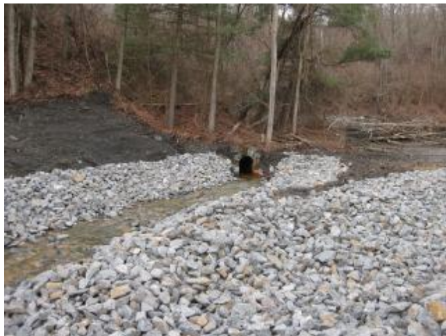
Rock-Lined Channel at Mine Outfall
