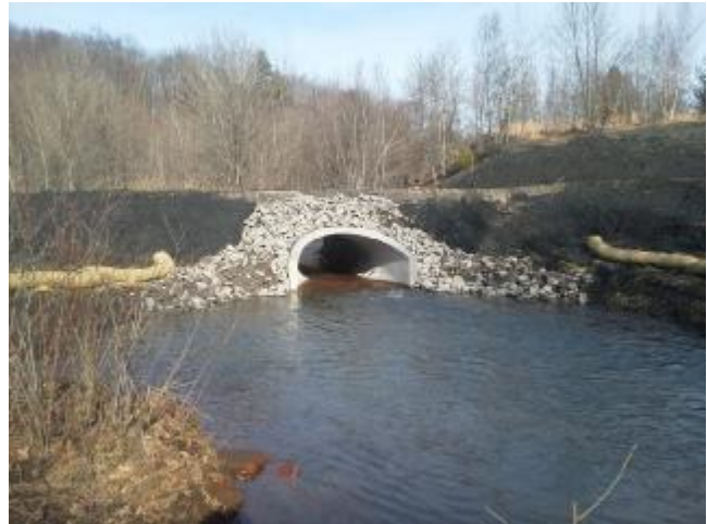
Replaced Haul Road Crossing
