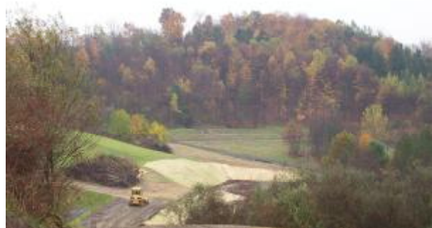
Site Overview and Vertical Flow Pond
