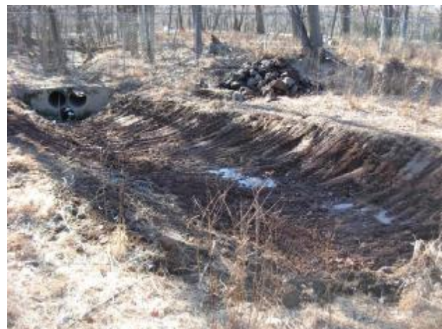
Drainage Swale after Remediation
