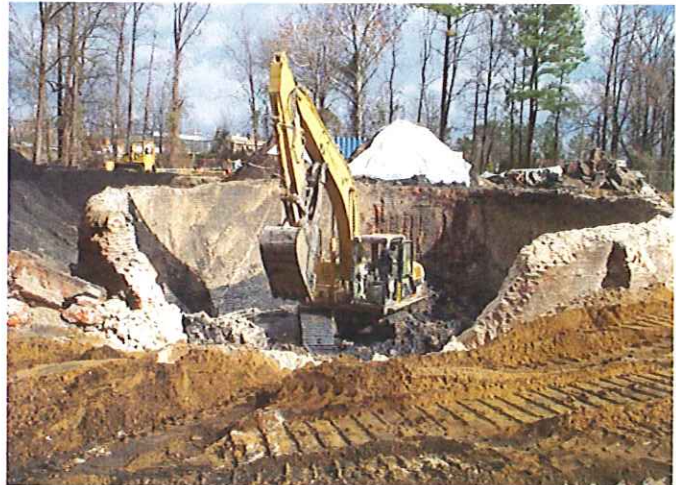
Gas Holder Demolition
