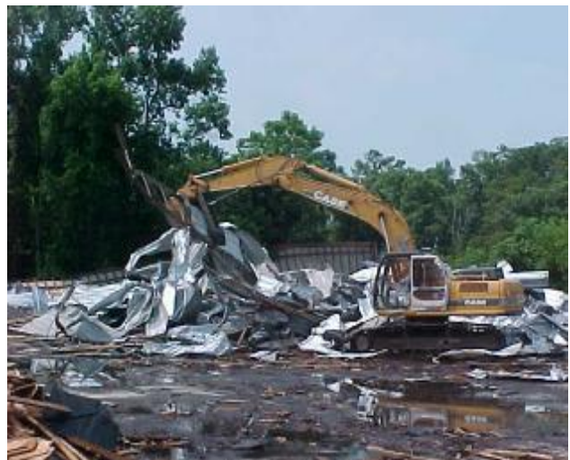
Warehouse during Demolition
