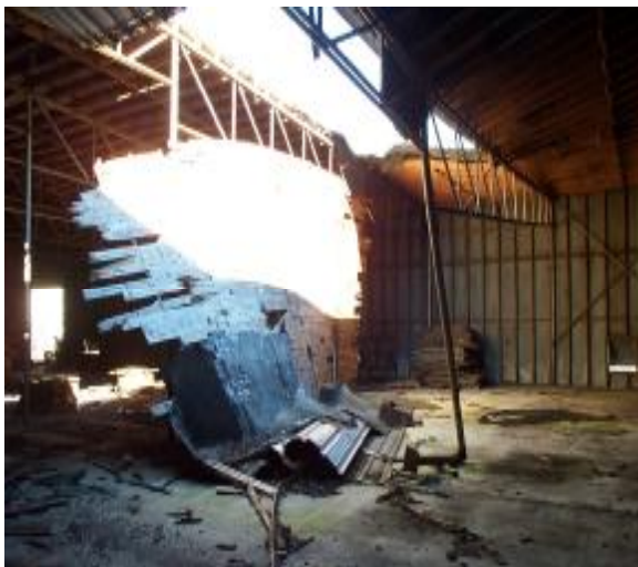
Original Condition of Warehouse
