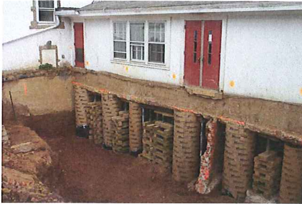
Installation of Temporary Supports and Permanent Concrete Piers
