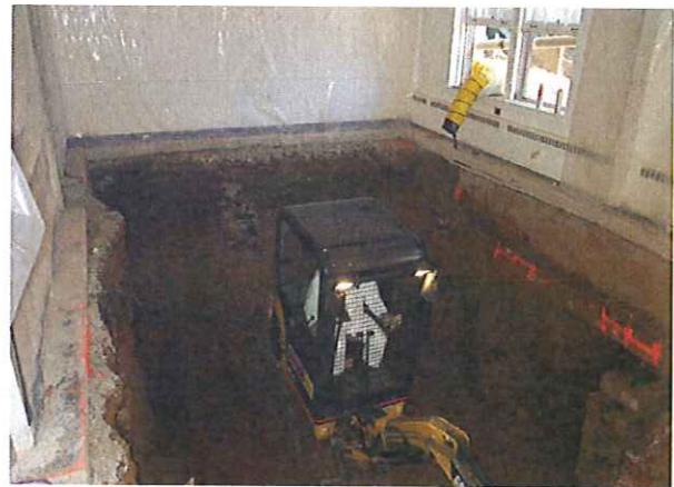
Excavating Underneath the Classroom
