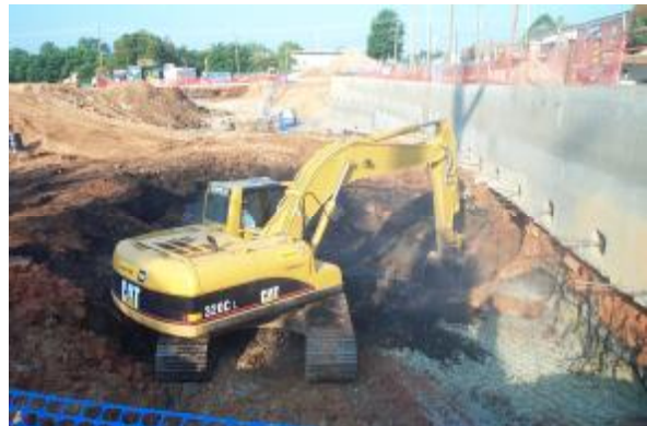
Secondary Holder Excavation
