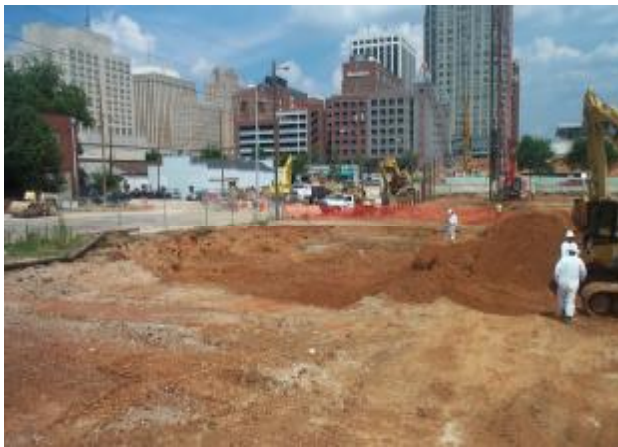
Initial Gas Holder Excavation
