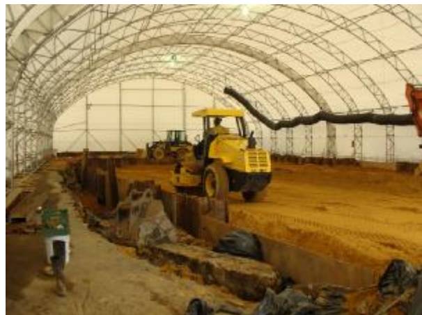
Backfilling Excavation Area
