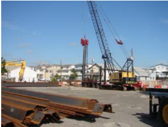
Installing Sheet Piling
