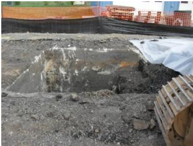
Excavation of Tar Separator Tank
