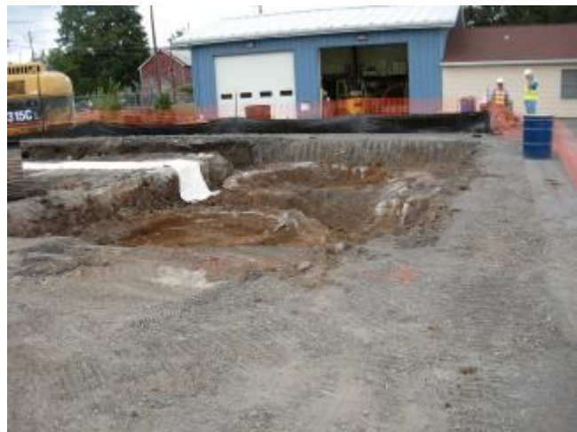
Surface Excavation of MGP-Impacted Soil
