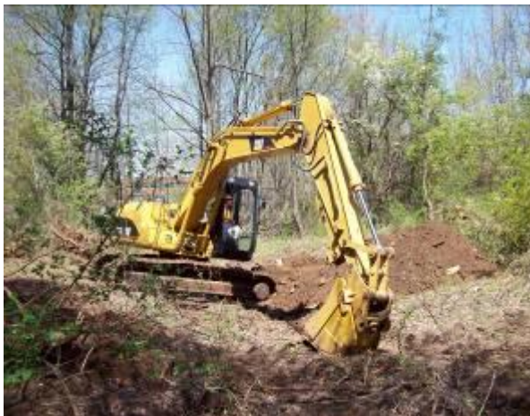
Test Pit Excavation
