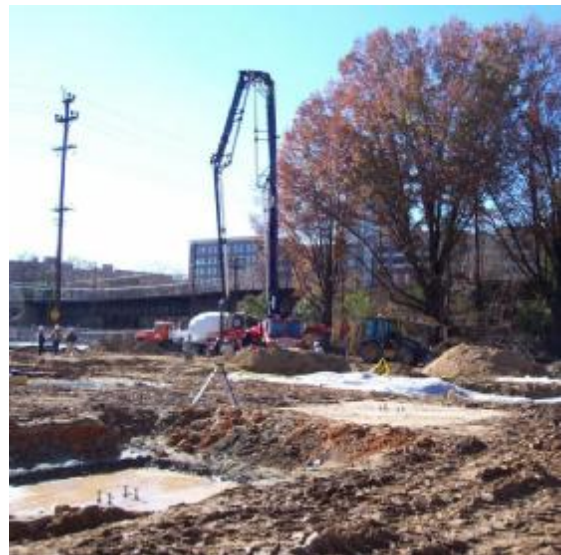
Concrete Placement Using 35m Concrete
