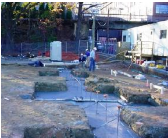
Perimeter Footers and Anchor Bolts
