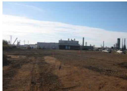
Final site grading
