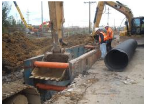
Using a trench box to install stormwater piping
