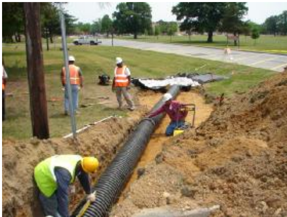
Stormwater Piping Installation
