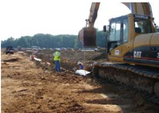
Sanitary Sewer Line Installation
