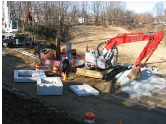
Setting Manhole Sections
