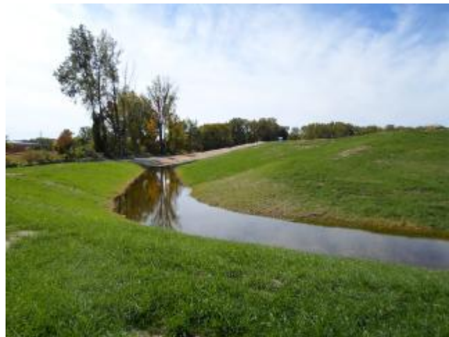
Completed Side Slope and Drainage Swale
