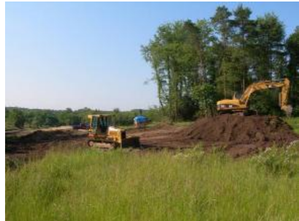
Stripping and Stockpiling of Topsoil
