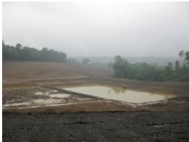
Construction of Permanent Pond
