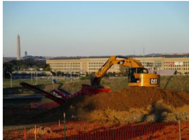
Excavation and Screening
