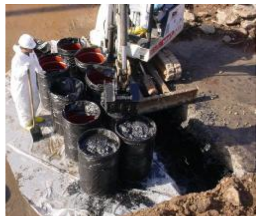
Coal Tar Removal
