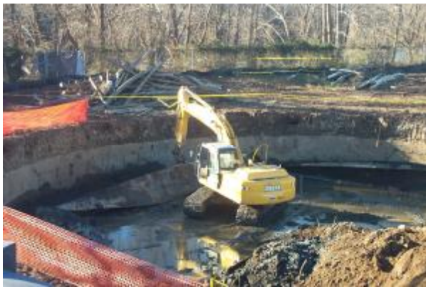
Gas Holder Remediation
