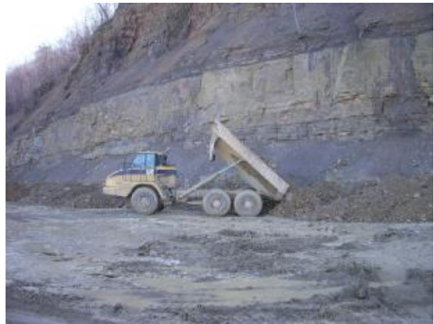
Backfilling the High Wall
