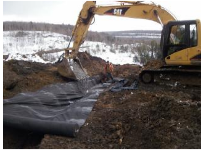
Installing Drainage Piping
