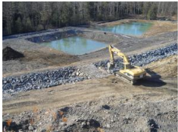
Construction of Treatment System
