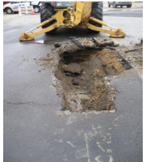
Excavation of 2,000-Gallon UST
