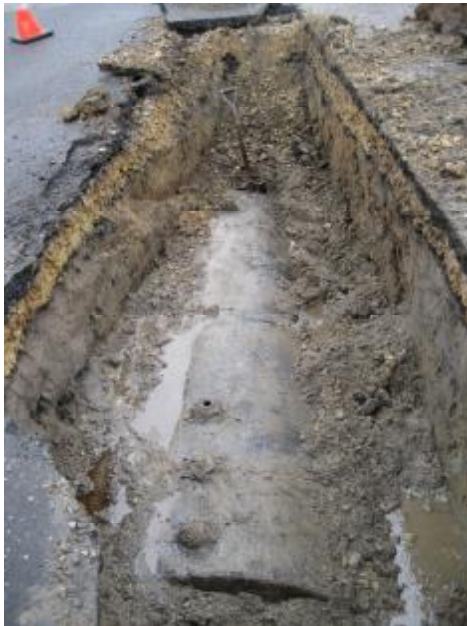
UST Previously Closed-In-Place
