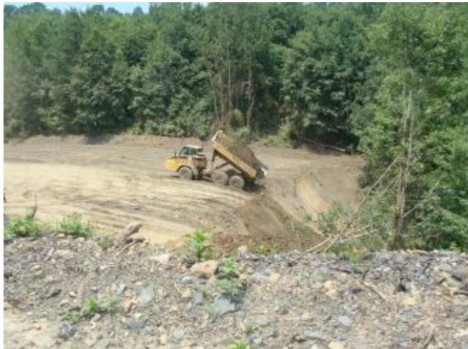
Relocating fill material via dump truck
