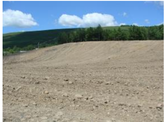
Finished graded area
