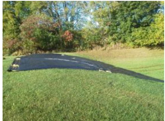
Berm Prepared for Stockpiled Soil
