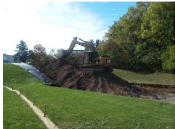
Load Out of Excavated Soil
