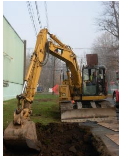
Excavating Contaminated Soil
