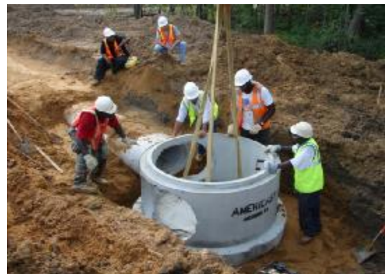
New Sanitary Sewer Manhole Installation
