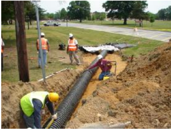
Stormwater Piping Installation
