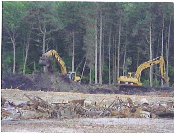
Excavation of Wetland Area Sediments
