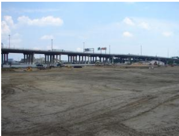
Placing Clean Fill Material
