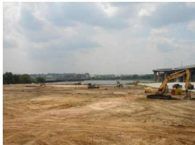
Placing Topsoil After Grading
