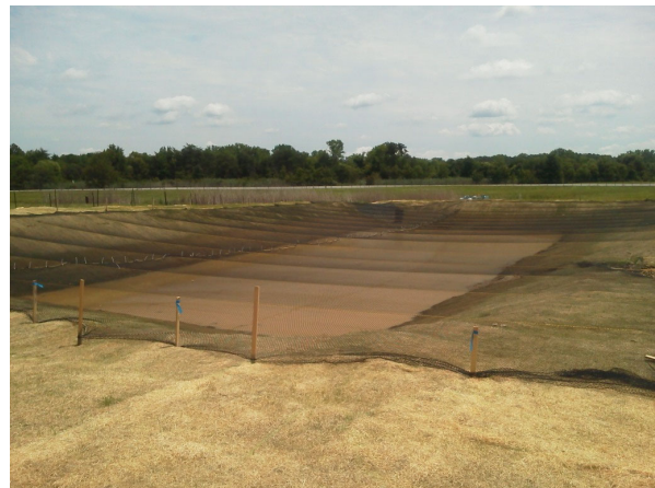
Sedimentation Basin with Bird Netting
