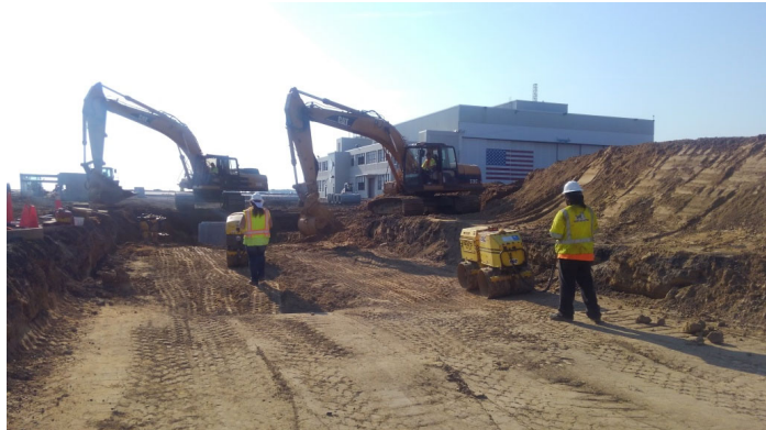
Backfill and Compaction
