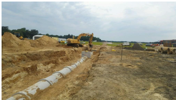
Installed RCP to Airfield-Rated Manhole
