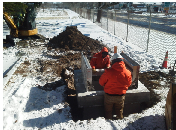
Installing New Well Vault
