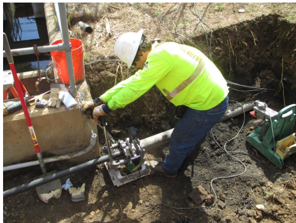
Fusion Welding Dual-Walled Piping
