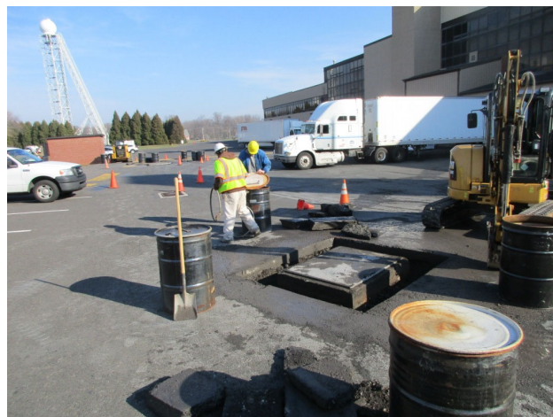
Replacement of Concrete Skirt around Vault
