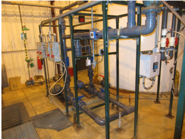
Replaced Piping and Pipe Supports
